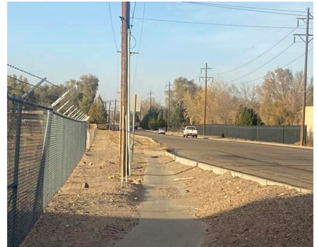
Overhead power lines and drainage
