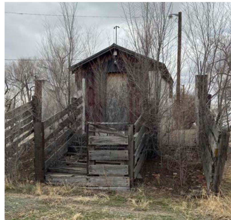
Former cattle chute
