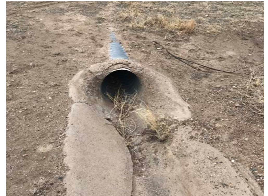
Shallow storm drainage on site
