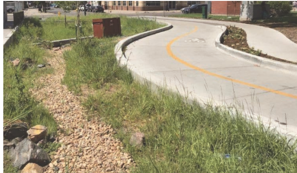
Example of stormwater swale for runoff
